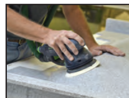
Final buffing and finishing onsite during installation
