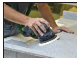
Final buffing and finishing onsite during installation
